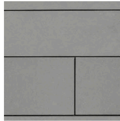
High-Density Fiber Cement Panel Rainscreen System [EQUITONE]
